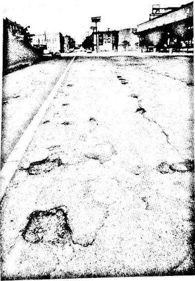
Freezing water expands, causing crevices in pavement to widen. Traffic turns the crevices into pot-holes.
